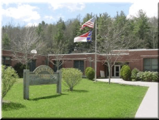
Macon County Schools, Franklin, North Carolina
